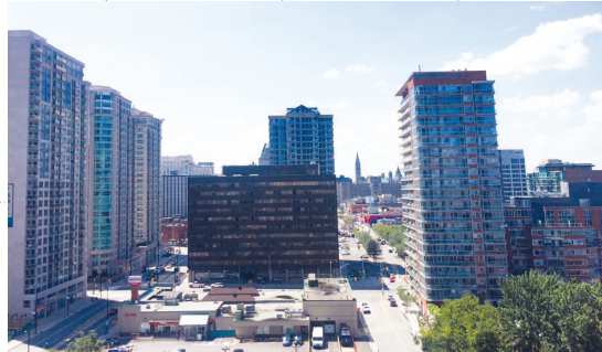
view to west towards Parliament Hill and neighbouring high-rise towers
